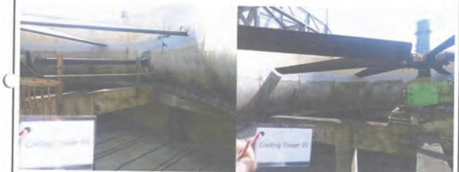
Fig. No. 2 Cooling cell 1 have many sediment, Clean by high pressure water jet.
